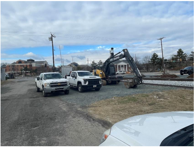
CSX equipment on site
