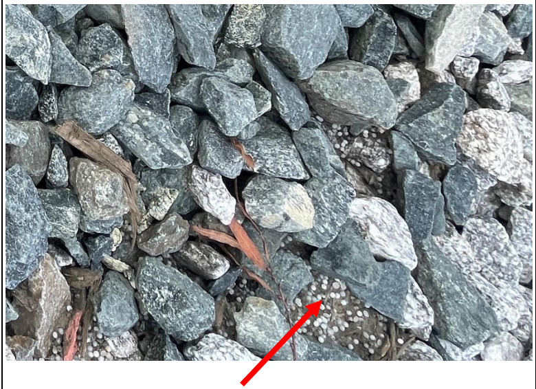
Close up of pellets along track in aggregate
