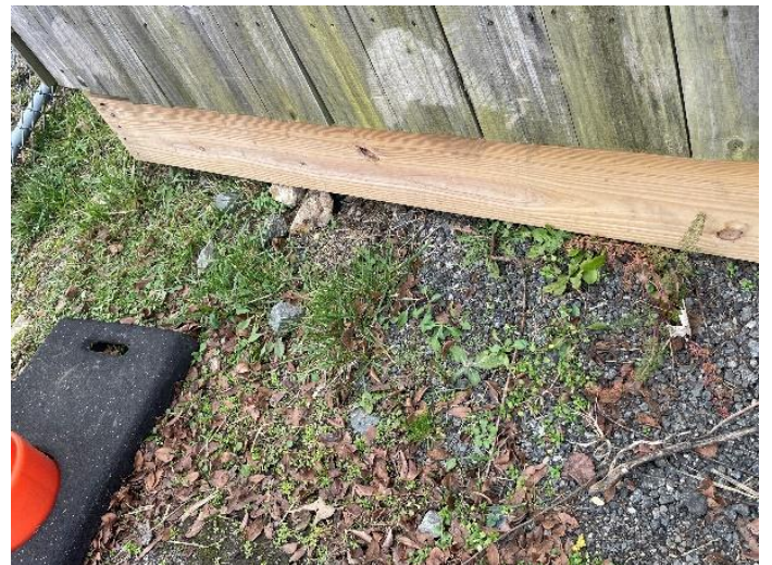
SE boarder pellets removed
